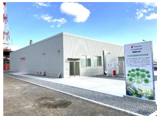
Bench-scale plant exterior
