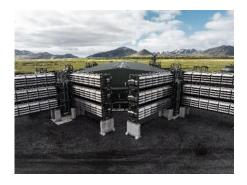
$Climeworks \ AG \ (Switzerland) \\ Operates the world's largest direct air capture (DAC) \\ facilities, "Mammoth," utilizing renewable energy to \\ remove \ CO_2 \ from the atmosphere and store it \\ underground.$
