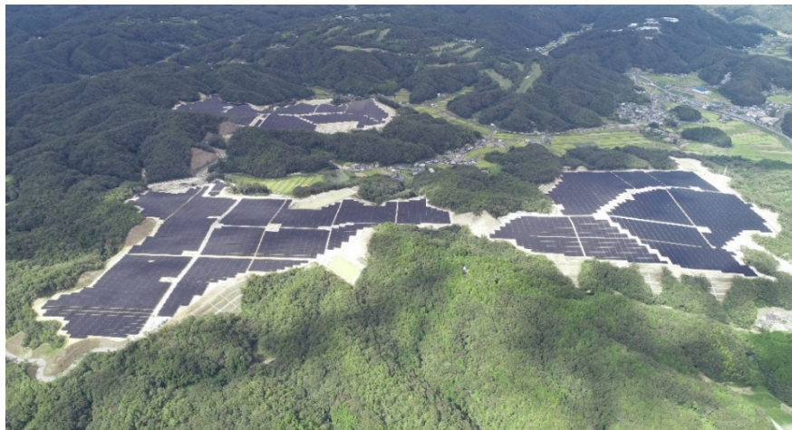
Panorama of SF Akaiwa Solar Power Plant
