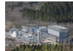
Takigami Binary Cycle Power Station
