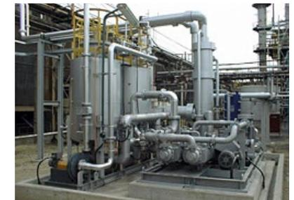
Exterior of IDESORB-B VOC processing equipment
